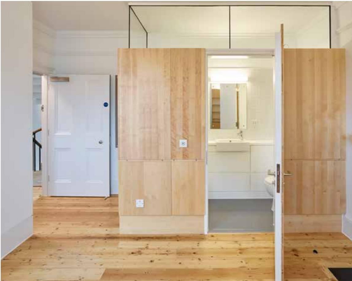
En-suites inserted into the existing floor plate bring 21st century amenity to a Grade I listed building. In order to avoid adding to the moisture load, shower rooms have been positioned away from external walls.
