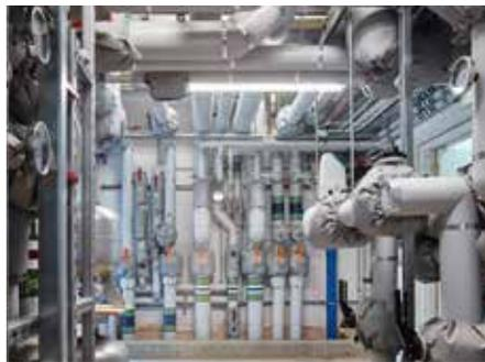
Left: A centralised plantroom efficiently provides heat and hot water and includes connections to the planned ground source heat pump.
