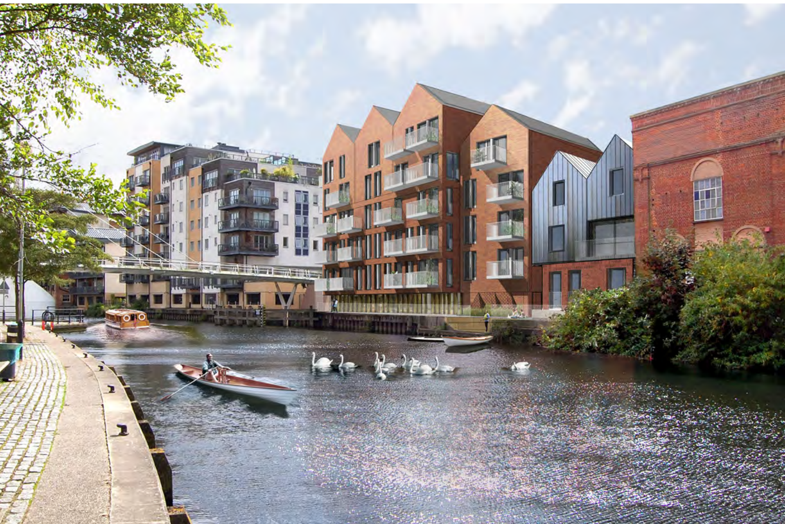
Below View from the opposite side of the River.
