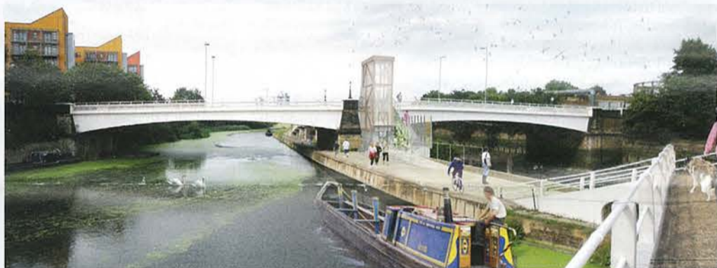
Twelvrees Bridge will contain a lift and staircase and link Three Mills with the eastern bank.
